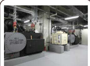
Setting a larger difference than before between the temperatures of cold and hot water which is the heat source of air conditioning reduced the power consumption of the water pump by decreasing the necessary amount of water.
