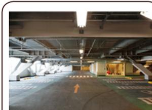
Ducts for ventilation of parking lots were eliminated and the circulation of air on each floor is facilitated by suitable positioning of small fans.
